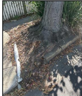
DAMAGE TO EXISTING STREETScape CAUSED BY TREE 32
