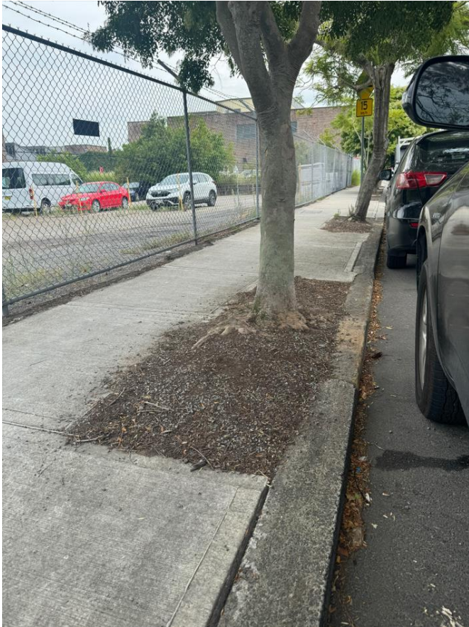
Figure 5 Tree 36 onwards (looking west), showing asphalt covering the gutter which will require regrading for compliance and water ingress
