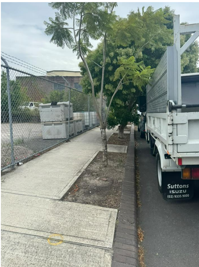
Figure 6 Existing brick paver kerb and asphalt laid over gutter
